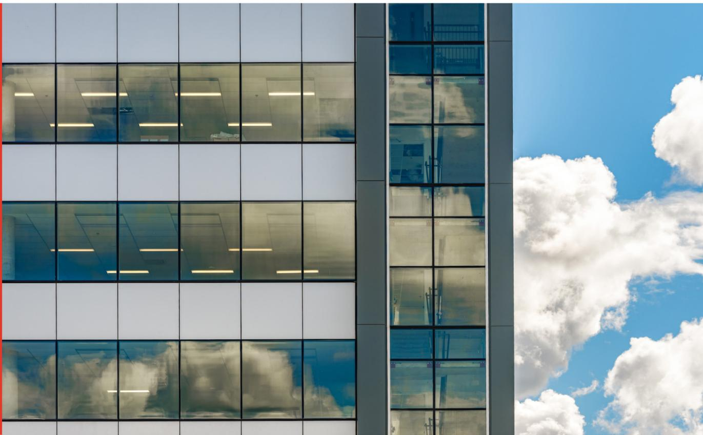
Kawneer's window wall and ribbon window solutions are designed to allow prefabricated, pre-glazed or site-glazed window and door units to be installed between the floor slabs of mid- to high-rise buildings in a variety of applications, giving the appearance of a curtain wall.
